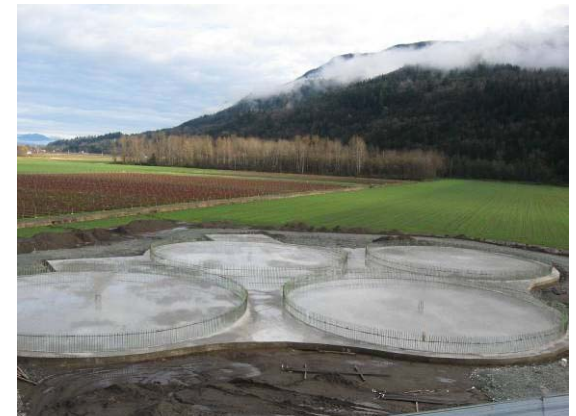
Catalyst Digester Pad – February 2010
