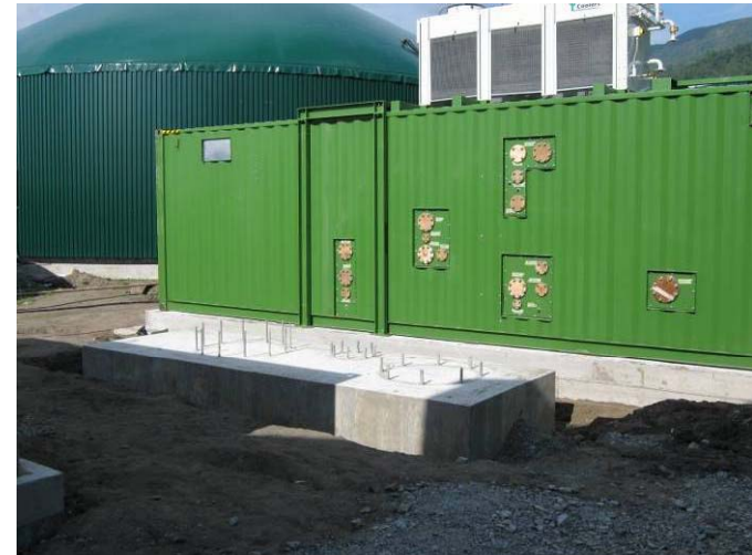
Greenlane Main Container Arrives – June 2010
