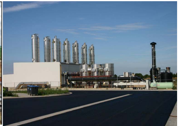
Greenlane® Biogas Upgrading Plant - Gustrow, Germany
