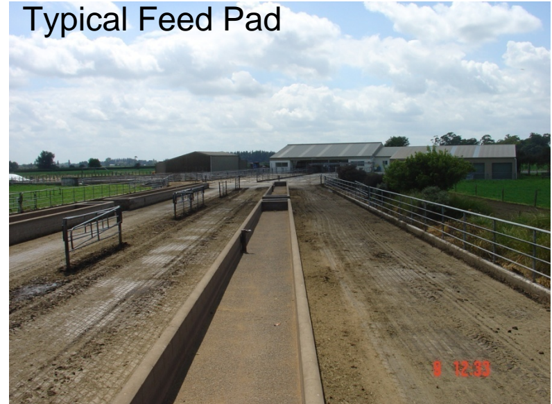
Typical Feed Pad Effluent Storage –emitting methane
