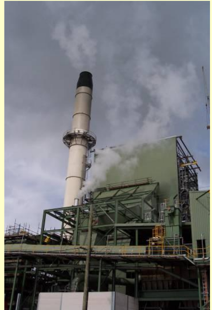
Condong Sugar Mill – NSW - 30 MW
