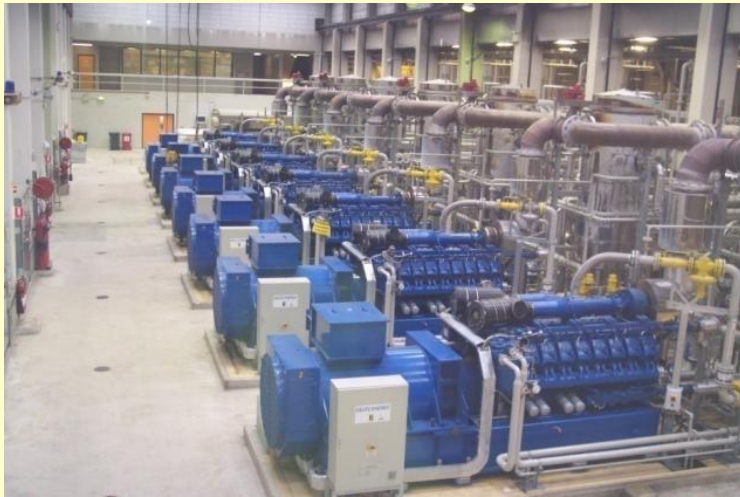
Carrum Downs Waste Water Treatment Plant, Melbourne
