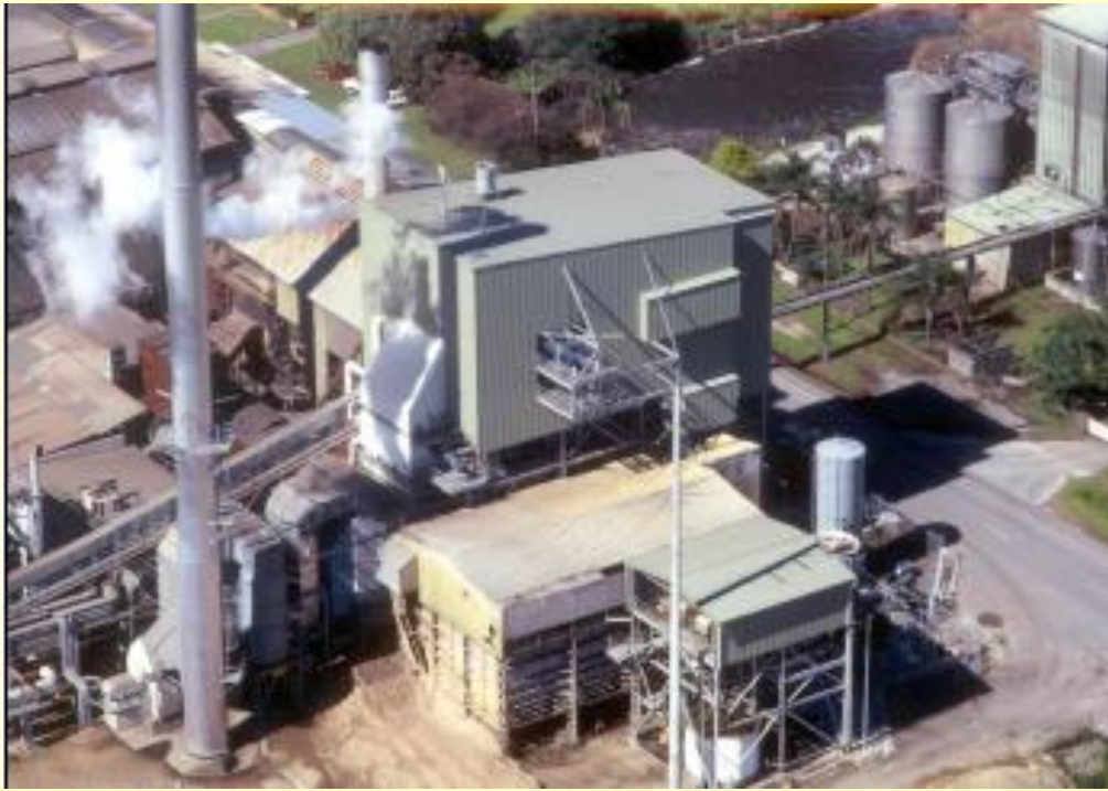
Rocky Point Sugar Mill – Qld -30 MW
