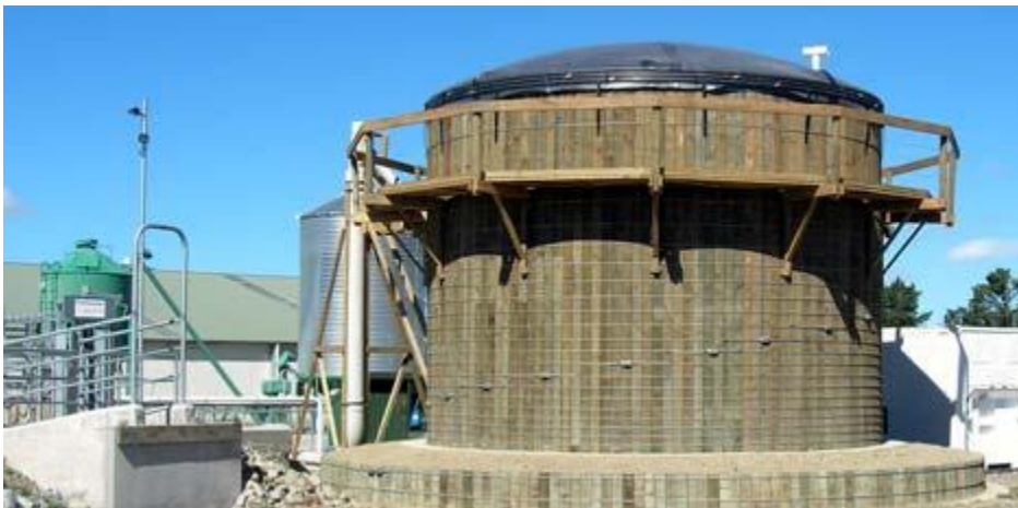
An AD digester in Canterbury uses dairy waste (courtesy Natural Systems Ltd)
