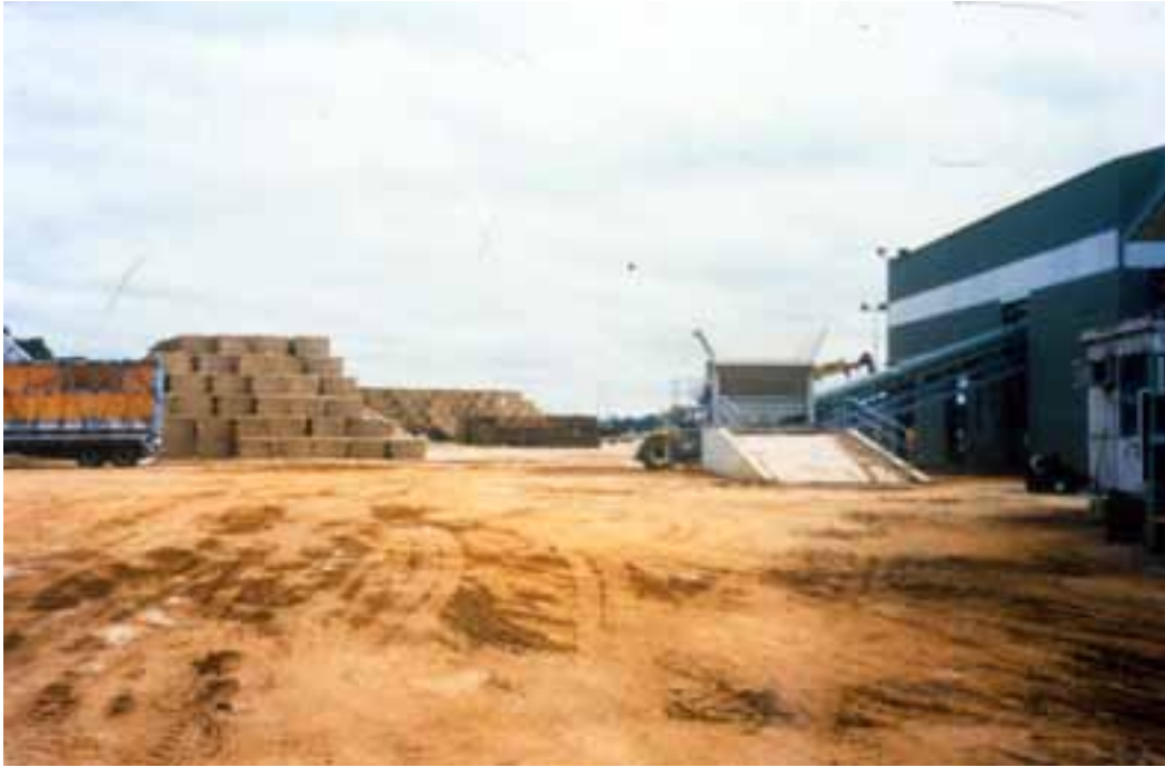
Figure 5-8: Bagasse baled and stored for use in a sugar processing co-generation plant during the non-cane crushing season
