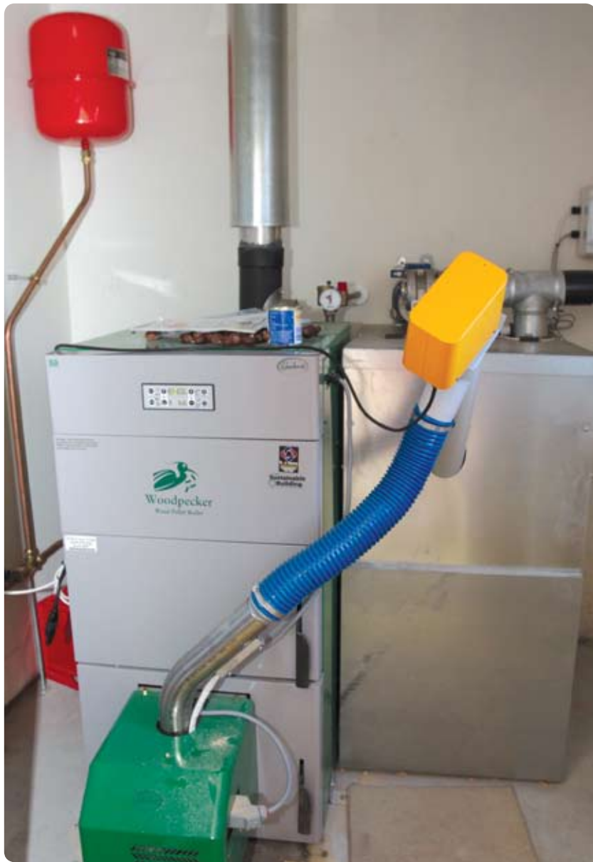
50 kW "Woodpecker" wood pellet-fired boiler.
