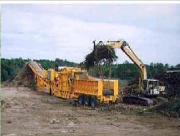
Figure 3 – Horizontal hogger with excavator loader
