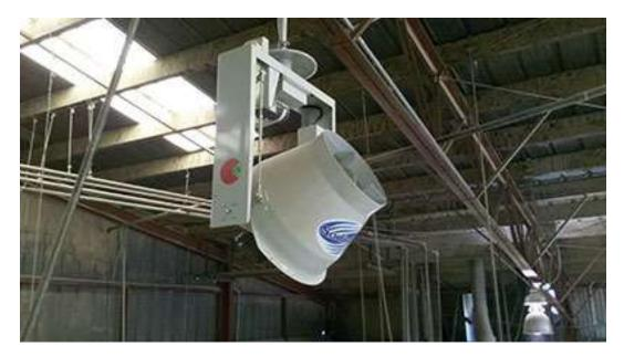
The SonicAire 2.0 installation in a planer mill prevents fugitive wood dust from accumulating by creating an overhead air curtain using BarrierAire Technology. Dust explosions are always a risk in any wood processing plant
