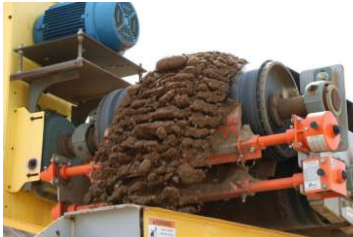
Belt conveyors move massive amounts of material, often at very high speeds
