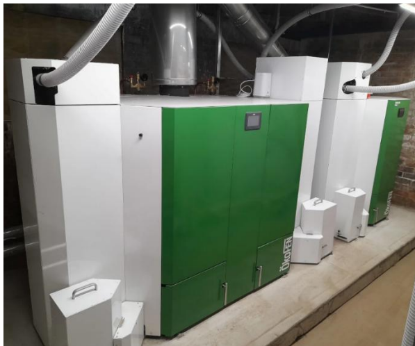
ÖkoFEN PES 128 and PES 64 Pellet Boiler Cascade System
