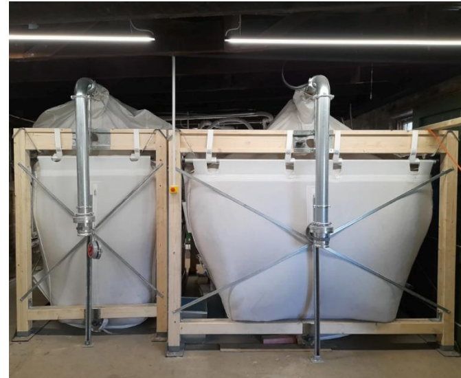
12 tonne capacity pellet hoppers with sloping floors
