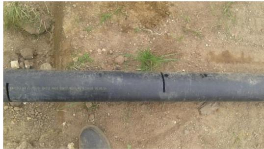
Figure 11: Perforated Pipe from Waikato Dairy Farm
