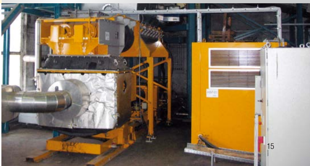
KOS 25100 with hydraulic power pack and twin-screw feeding device, transporting biomass to the fermentation tank
