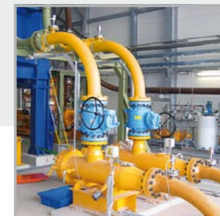
Left: Retained foreign bodies Right: Foreign body separator in a power plant
