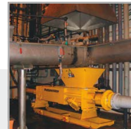
Pumping screenings (Coney Island, New York)
