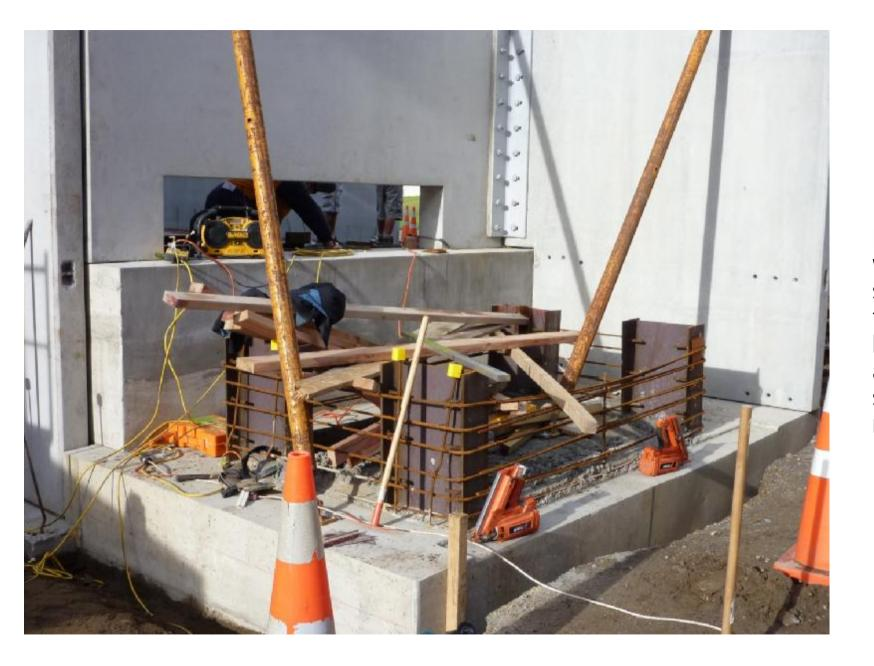
No complex civils work is required, such as this plinth for the cast-in hydraulic ram anchor, and the suspended wall for material discharge.
