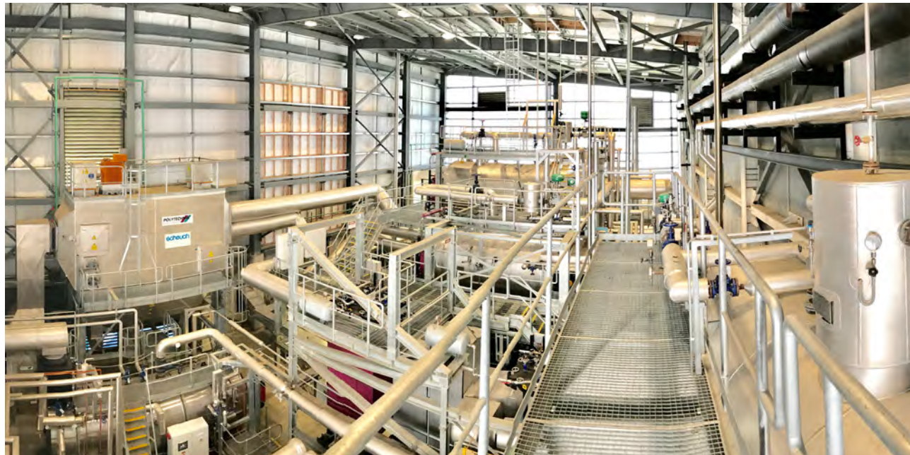
CLOCKWISE FROM TOP: Nelson Forests sawmill near Blenheim; Burwood Hospital Christchurch. Photos: Polytechnik Biomass Energy New Zealand.
