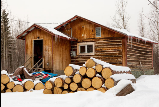
A typical site in Koyukuk. Logs cut in 4-foot lengths sized to fit trailers and sleds. The logs will dry out for a year, and be cut and split into firewood when needed.
