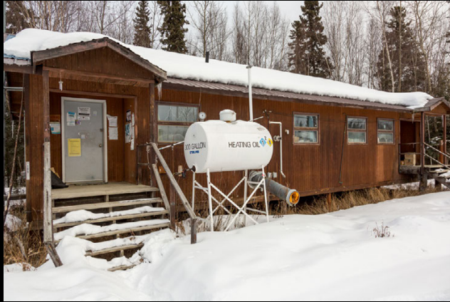
Koyukuk's library heats almost exclusively with heating oil. A wood stove could heat this small building, but someone would need to stoke it in the middle of the night so that the library could be used first thing in the morning.
