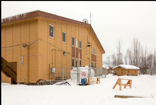
The Ella B. Verneti School is heated with both heating oil and recovered heat from the adjacent power plant. It is difficult to imagine heating this 13,896 sq. ft. building with conventional wood stoves.
