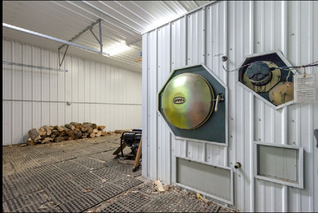
Koyukuk's biomass heating plant is a separate building located near most of the village's community buildings. The messy part of heating with wood stays here.
