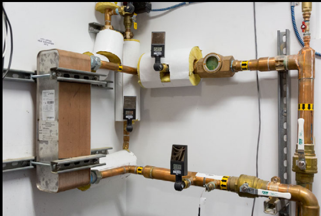
This is all it takes to connect a building's existing heating system to the biomass heating plant: this small heat exchanger (left) and two heat distribution pipes (right).
