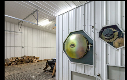
Biomass Heating Plant
