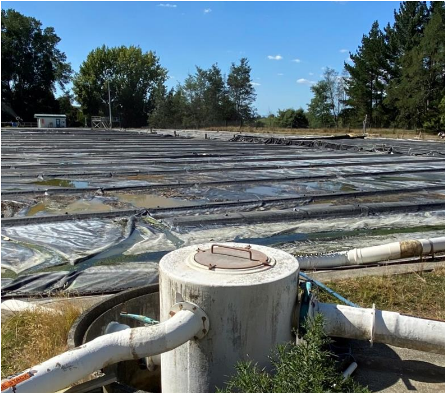
Figure 5: Fonterra's Tirau Anaerobic Lagoon Digestion Plant
