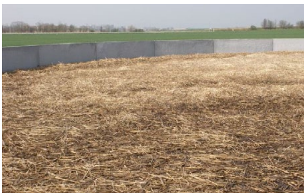
Figure 12: Example of Permeable Constructed Cover 37
