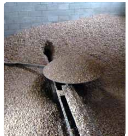
Fuel storage bunker
