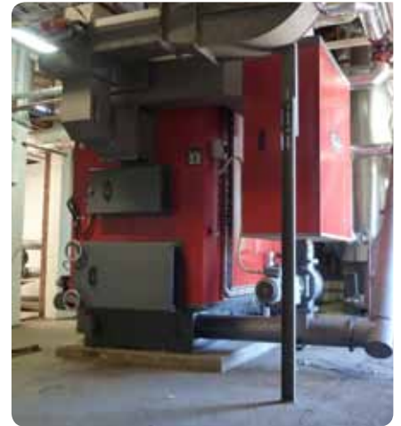
The boiler at LSP
