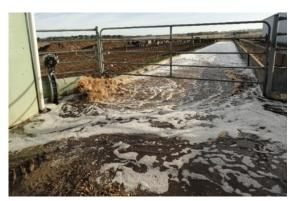
Figure 3-1: Typical dairy effluent systems used on-farm in Australia, showing a flush tank being used for flushing of a dairy feed pad area. Photo courtesy of Dr. Scott Birchall and Dairy Australia.
