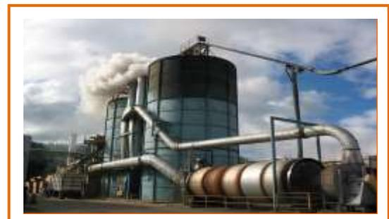
The unit burned all the dry shavings also produced on site and a proportion of the wet sawdust produced. There was a limit to the quantity of wet sawdust which could be burned due to the furnace grate configuration.
