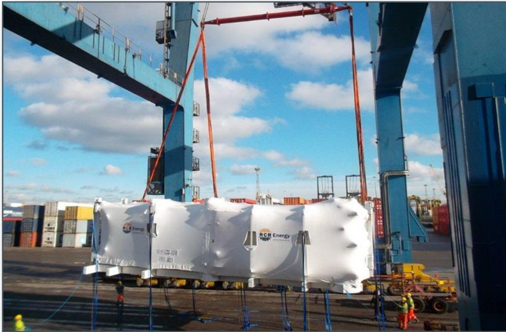
Boiler unloading at Tilbury Port, UK
