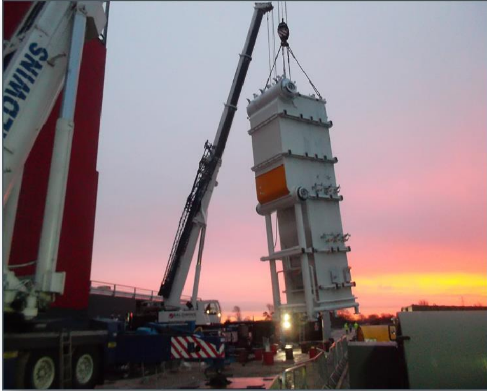
Lifting into position at site, Tutbury UK
