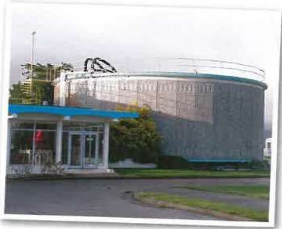
Digesters upgraded by Calibre Consulting for Palmerston North City Council's wastewater treatment plant.
