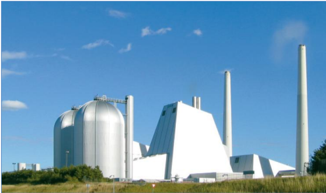
Figure 11: Two pressurised 22,000 m 3 heat accumulators at Avedøre Power Station in Copenhagen, capable of storing 8000 GJ of heat (Petersen and Aagaard, 2004)
