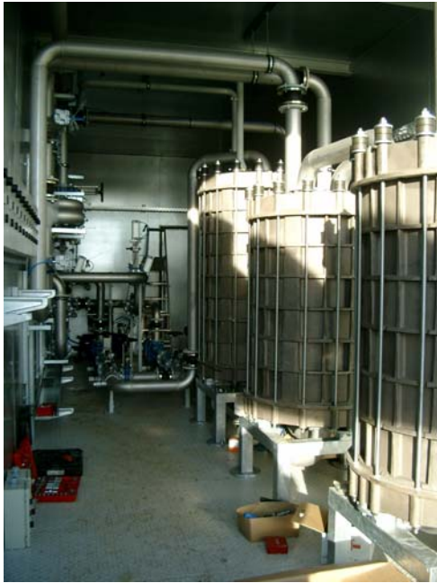
Figure 1: Example of a containerised module for pasteurisation of 100 t/day of incoming liquid waste in a digester facility.
