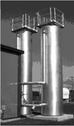
Picture 3: Sulfatreat® H 2 S-removal
