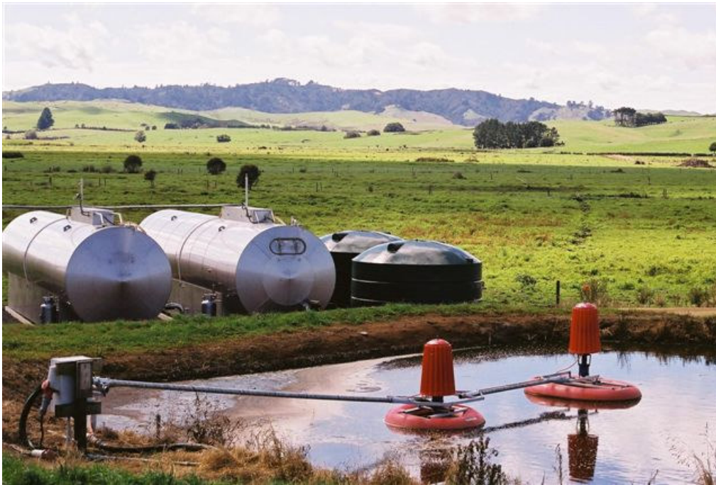
Figure 3. Two of Three ISE Digesters Producing Bacteria-Free Fertiliser and Methane Gas at Orini Downs Dairy Farm
