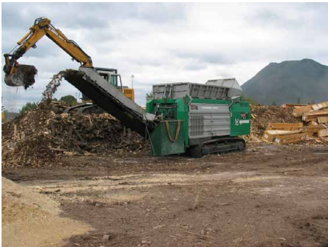
Figure 5 - Materials Processing's Crambo 6000 turning stem off-cuts, bark and packaging waste into boiler fuel (see Appendix III)
