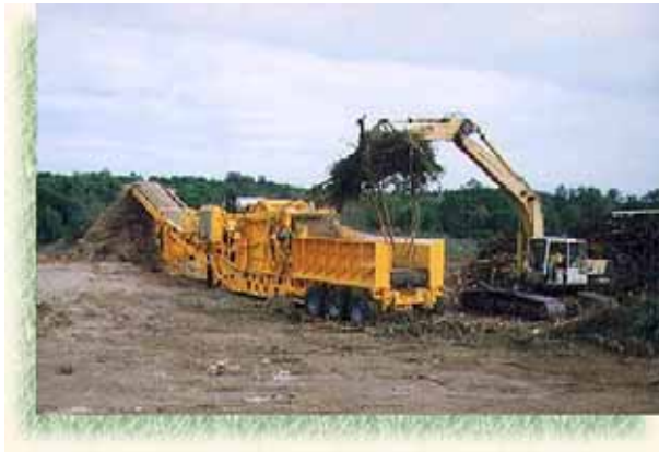
Figure 9 – Horizontal hogger with excavator loader
