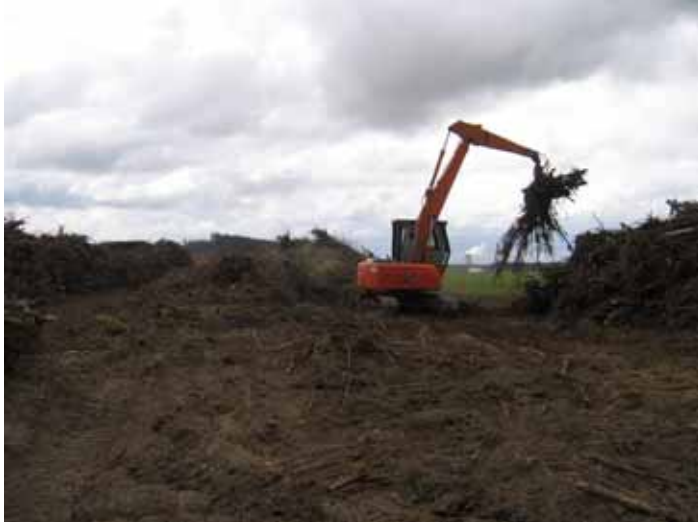
Figure I-4 – Excavator pre-treating windrows, one windrow is piled into two rows for feeding into the Ripper.
