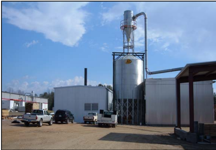
Figure 9. Typical Advanced Recycling Equipment (ARE) combustion facility with silo storage. 57
