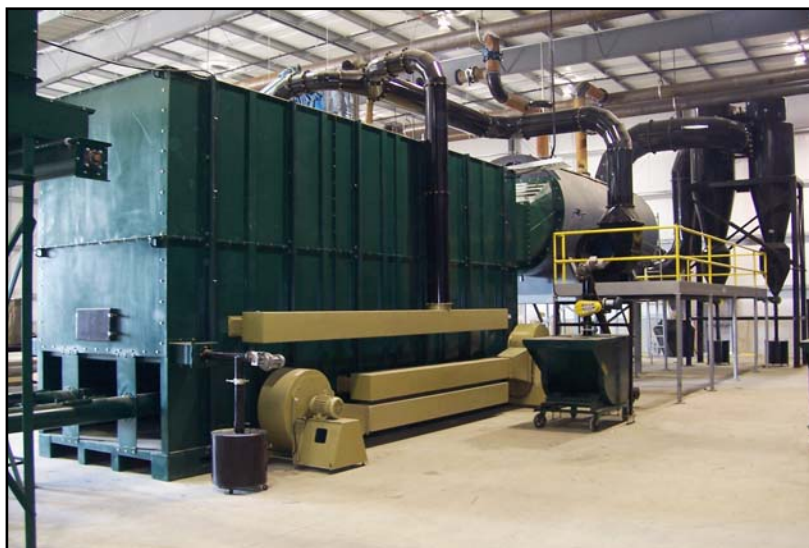
Figure 5. Typical combustion unit for a “hot water” system provided by Advanced Recycling Equipment (ARE). 27
