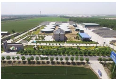
The biogas and biomethane plant in Dingzhou, China produces 400 Nm<sup>3</sup> per hour of biomethane for the transport sector
