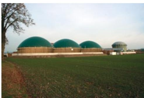
Waste digestion plant (1 MW<sub>el</sub>) with an input of 24,000 t per year
