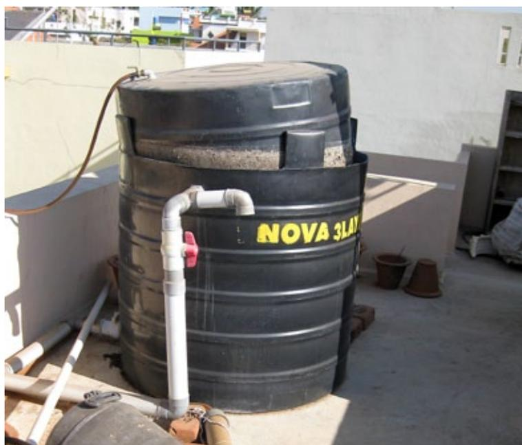
*Producing biogas in a domestic digester*
