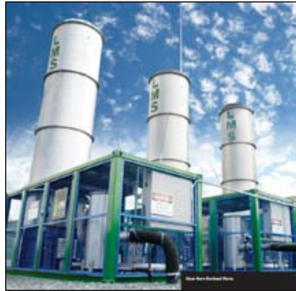
Figure 2: Enclosed flares with containerised auxiliaries
