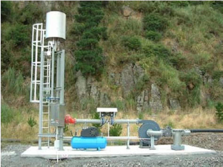
Figure 9: Open flare with knock-out pot, flow meter, fan, air operated shut down valves (2), air compressor and flame arrestor (red)
