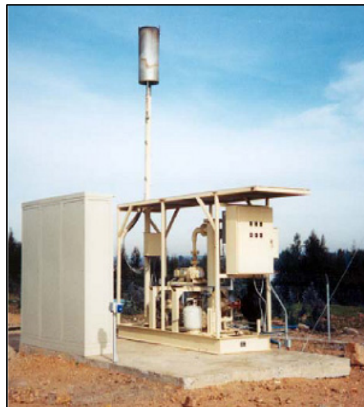
Figure 3: Open flare with blower, control panel and electrical cabinet in the foreground
