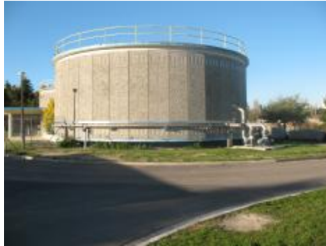
New External Mixing System on Digester 2
