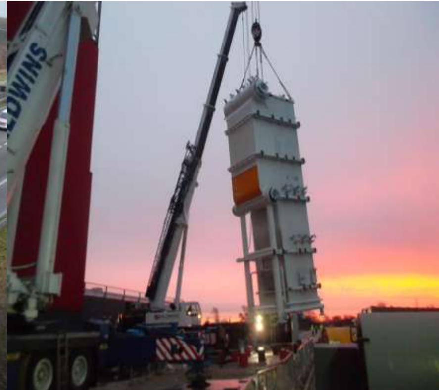
9MW Coffee Waste Fired BFB Boiler – Nestlé UK 1 Piece Shipping & Erection
