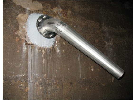
Close up of SS injector
