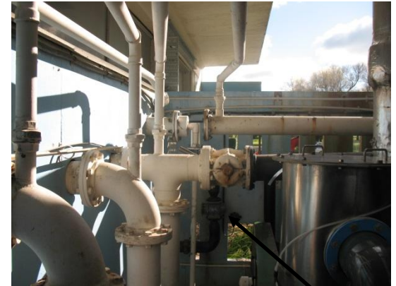
Undersized flow meter
