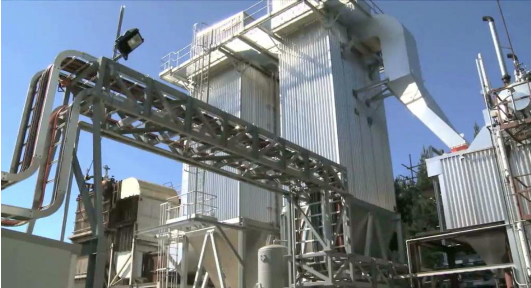
10 MW Wood Chip and Residue Boiler
