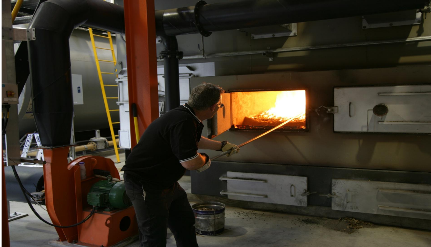
4 MW Seasoned Wood Chip Boiler
