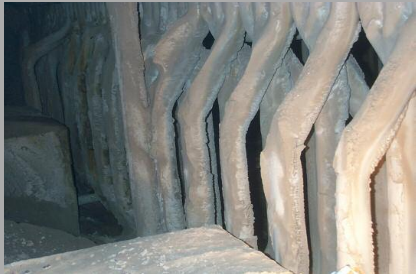
Boiler exit screen – 76mm O.D. tubes
