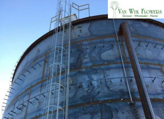
2ML heat store; part of thermal design, load buffering, peak power delivery
