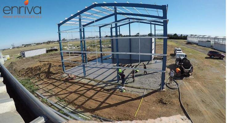
Completion of concrete works in plant room Steel anchors tied into the concrete, imperative for the live floor loads
